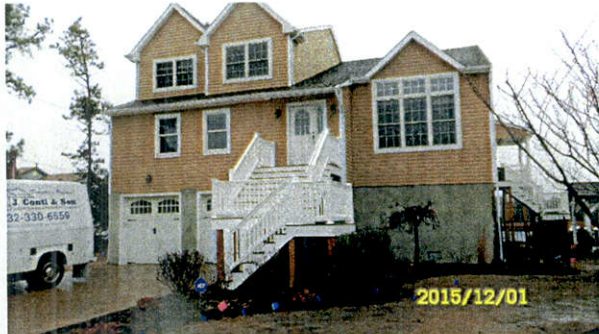
FRONT OF 34 KETTLE CREEK DRIVE
