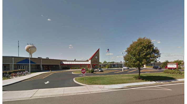
Ventnor Educational Community Complex (VECC)
