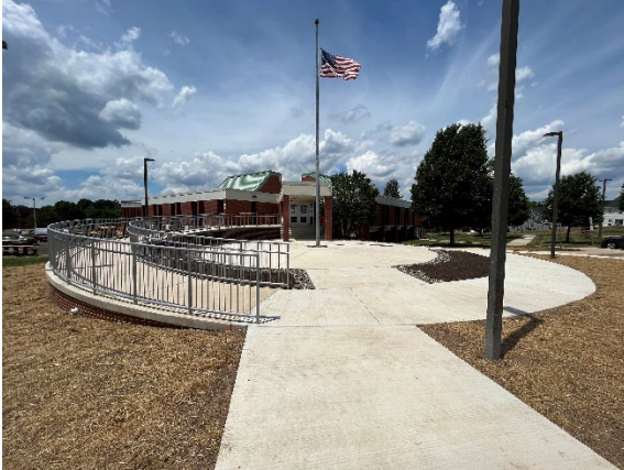
Administration Building ADA Ramp Improvements, Norristown Area School District, Norristown, PA
