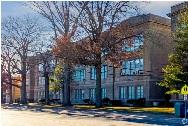
Middle School Façade Repairs, Hackensack Public Schools, Hackensack, NJ
