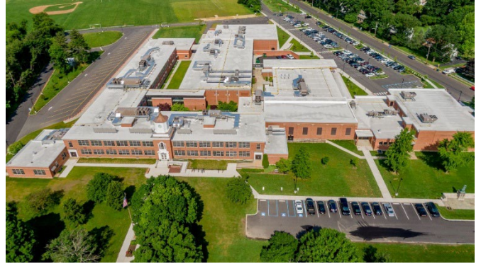
Pennwood Middle School Renovation, Pennsbury School District, Yardley, PA
