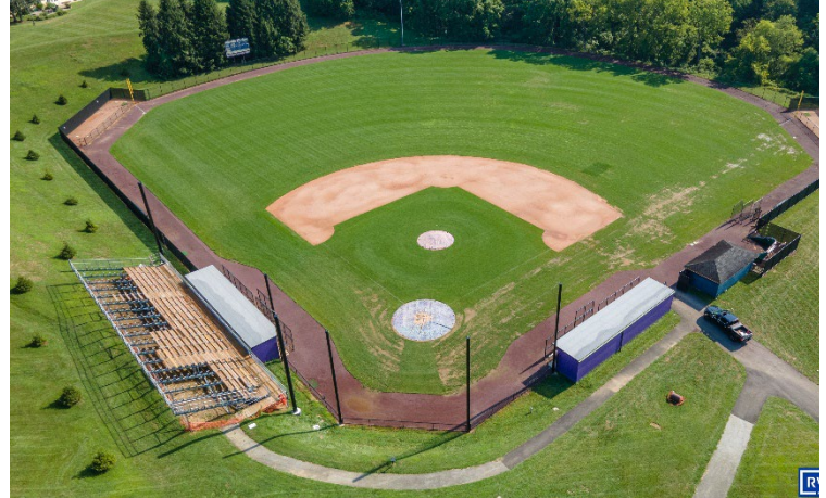
Serpico Stadium Improvements, West Chester, PA
