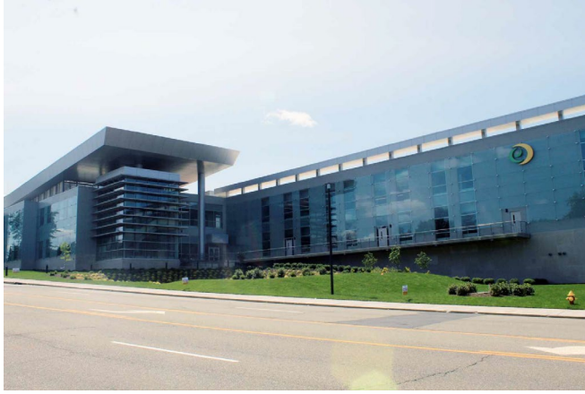
New West Caldwell Campus at Essex County College, West Caldwell, NJ
