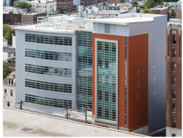
New STEM Building, Hudson County Community College, Jersey City, NJ
