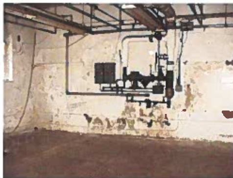
Basement Level - "Before"
