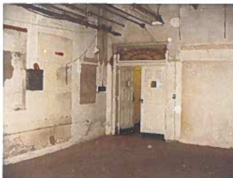
Basement Level - "Before"
