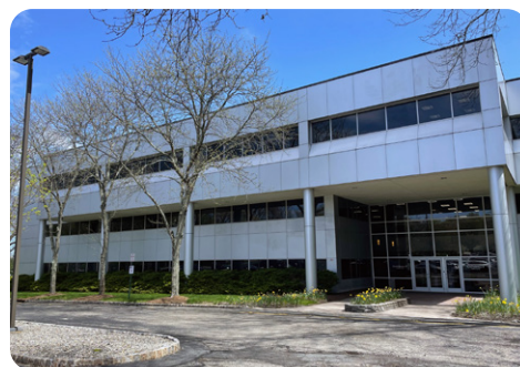
One Gatehall Drive Parsippany, NJ
