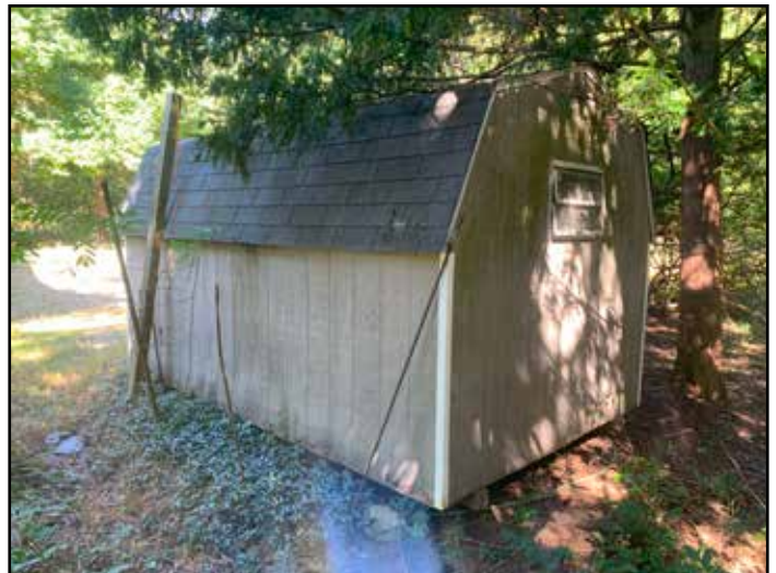
Figure 40: View of shed in side yard.
