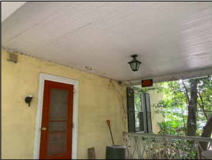
Figure 37: View of vacant Lutkins house front porch.
