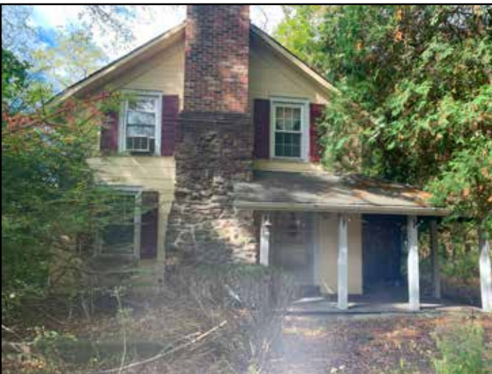
Figure 21: Vacant Mill House front facade
