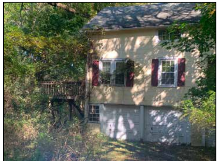
Figure 22: Vacant Mill House side facade with overgrowth.
