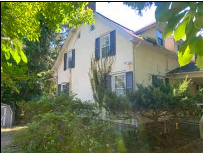
Figure 39: View of vacant Lutkins house side facade with overgrowth.
