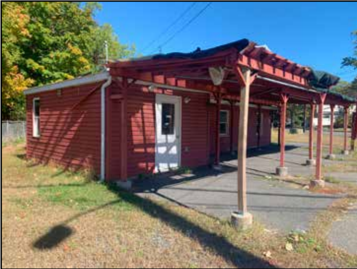
Figure 7: Vacant former garden center commercial building looking north.
