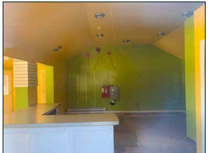
Figure 18: View of interior of the vacant former garden center with exposed concrete floors.
