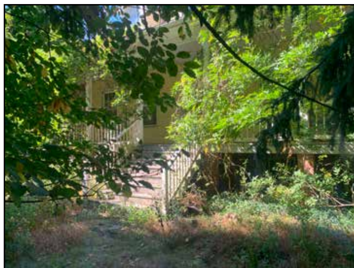
Figure 34: Vacant Lutkins house rear porch with overgrowth.
