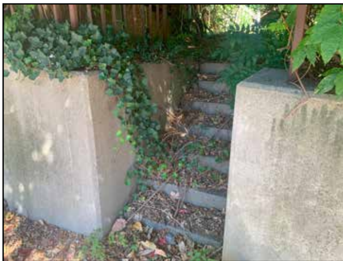
Figure 59: View of the retaining wall and stairs from West Ridge-wood Avenue
