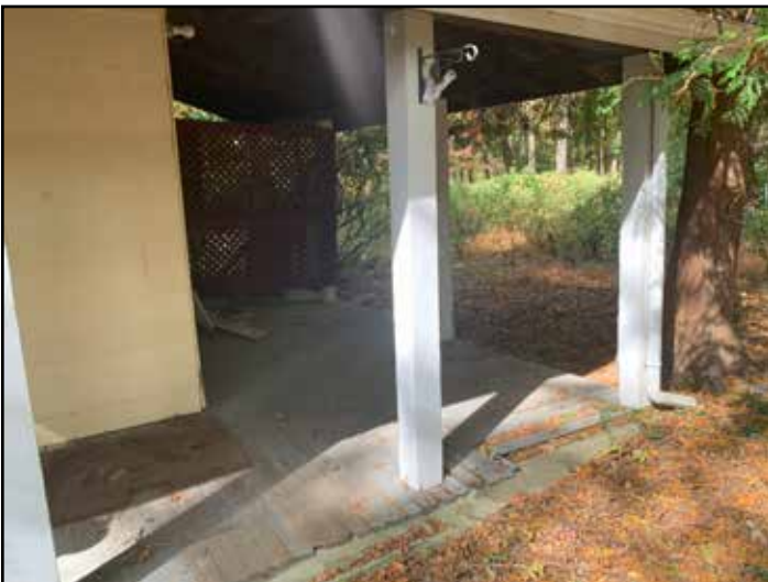
Figure 27: Vacant Mill House front covered porch
