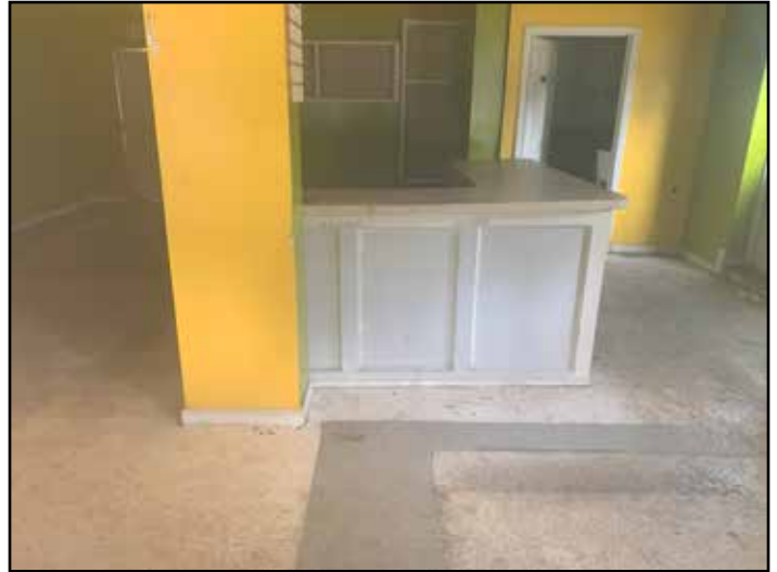
Figure 14: View of interior of the vacant former garden center with exposed concrete floors.
