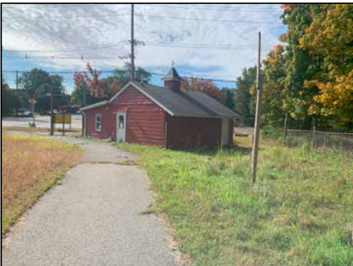
Figure 11: Vacant former garden center commercial building looking north.
