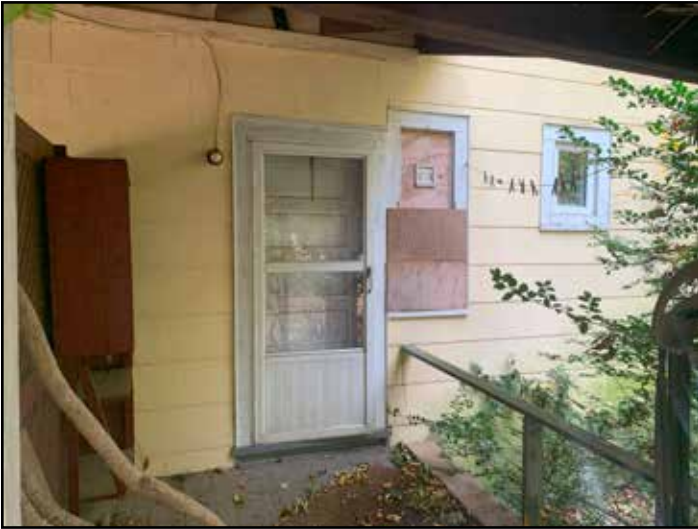
Figure 25: Vacant Mill House side door with bordered window.
