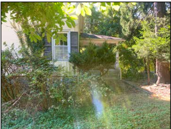
Figure 35: Vacant Lutkins house front porch with overgrowth.
