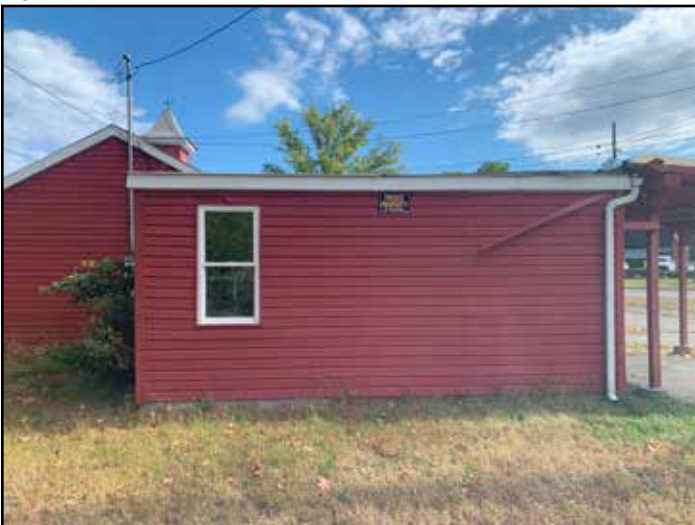
Figure 9: Vacant former garden center commercial building looking north.
