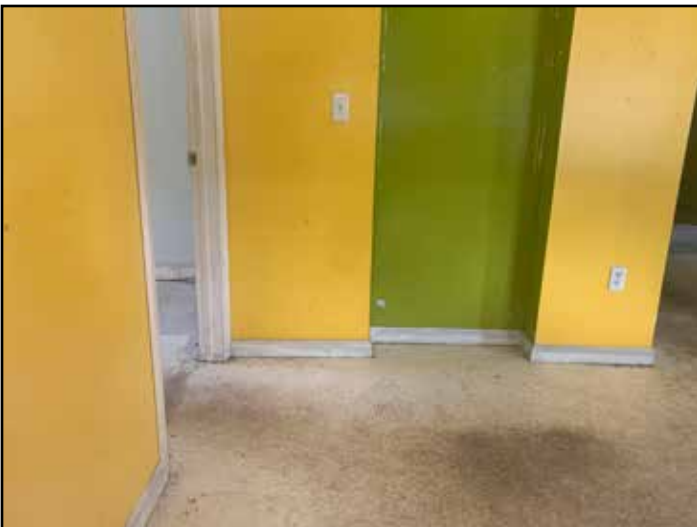
Figure 15: View of interior of the vacant former garden center with exposed concrete floors.
