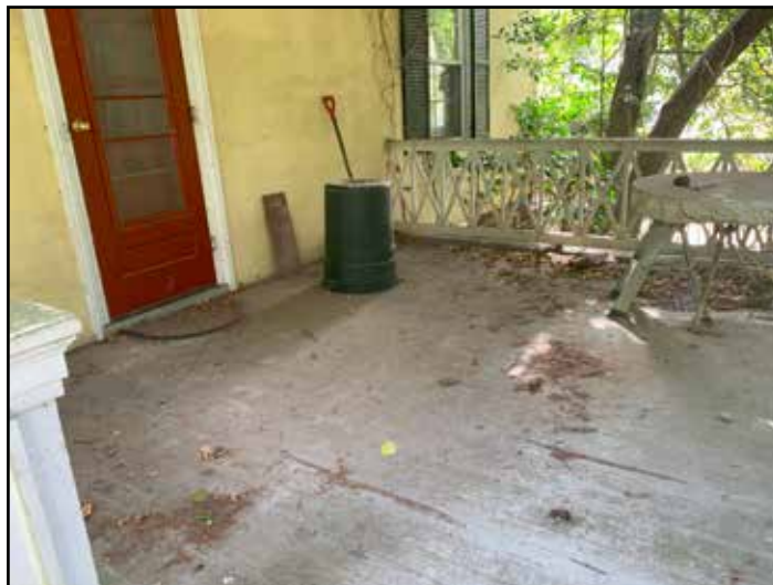
Figure 36: View of vacant Lutkins house front porch.
