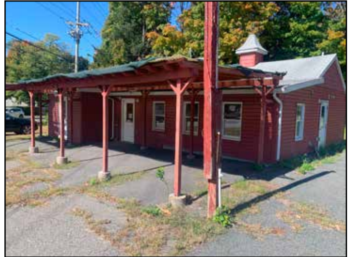
Figure 8: Vacant former garden center commercial building looking south.
