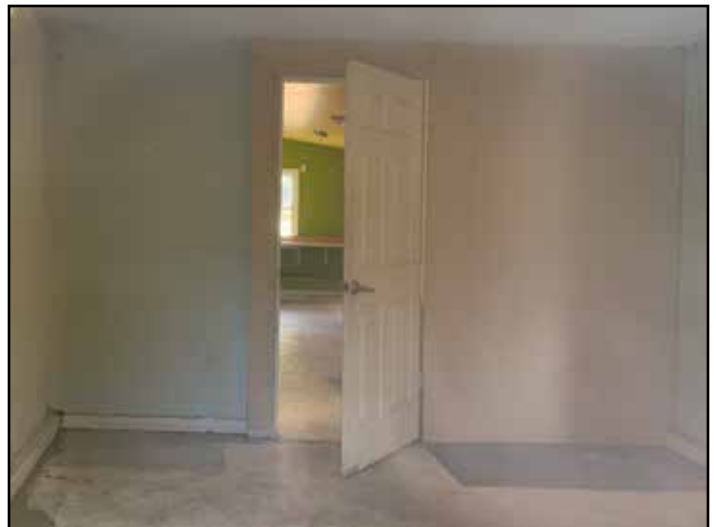
Figure 16: View of interior of the vacant former garden center with exposed concrete floors.
